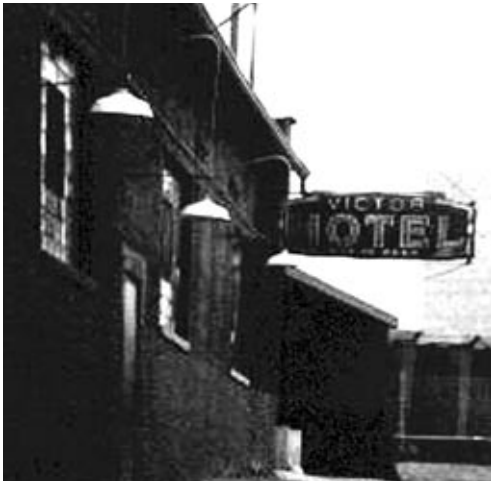
Shelter before demolition in the new millennium
